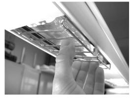
3) Remove new lamp from packaging and grip around large diameter of ceramic end. Insert alternate end of lamp into ceramic terminal block, taking care to line up Center Boss of lamp, with terminal Pin in terminal block.
